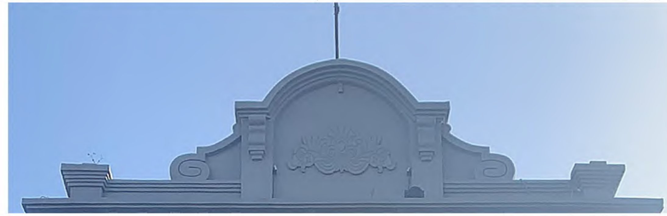
4.北側沿街立面屋顶装饰
