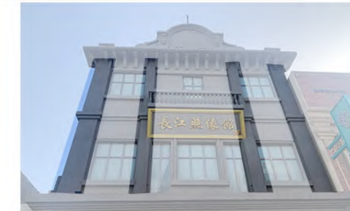
5.北側沿街立面扶壁柱
